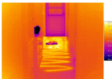
Varmekabler under fliser.
